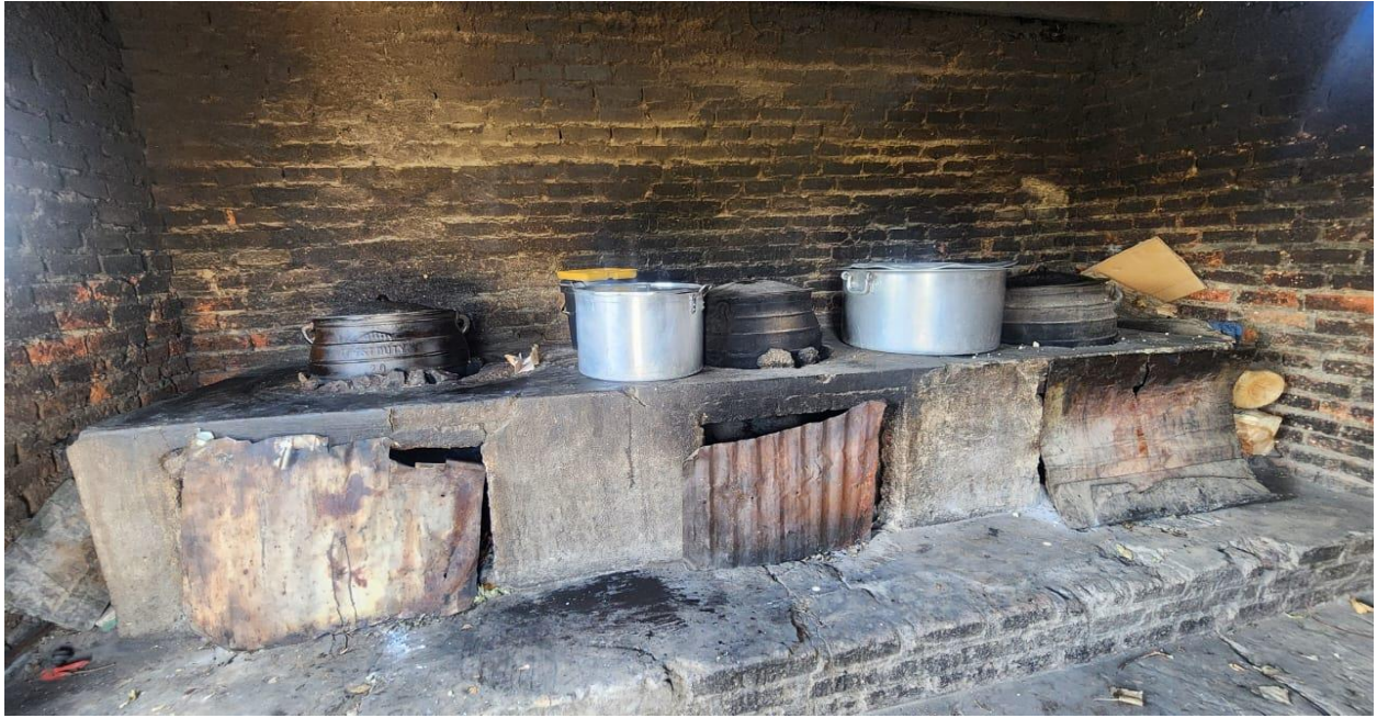
Figure 5: Lepereng Correctional Facility Cooking Area
